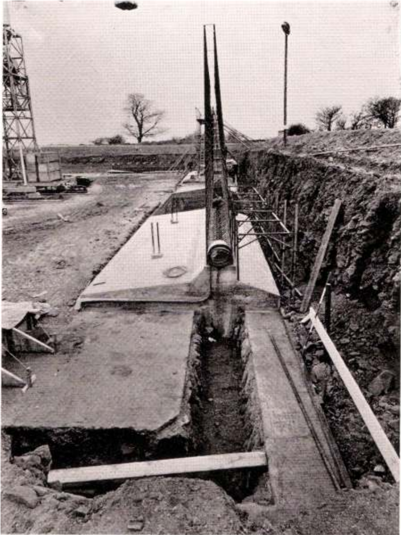
Crich Reservoir - Wall footing during construction
